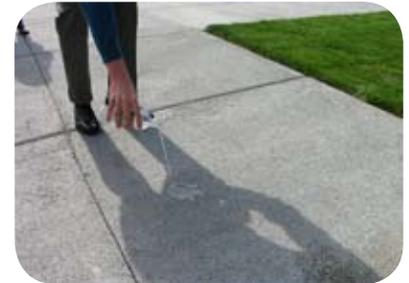
**Permeable interlocking concrete pavers** are similar to regular pavers except they are installed with wider joints or openings at the corners, allowing rainwater to drain into the joints between the pavers and down through an open-graded base. Most commonly used for parking lots and walkways, these interlocking pavers provide a surface that is stable enough for vehicular traffic.
