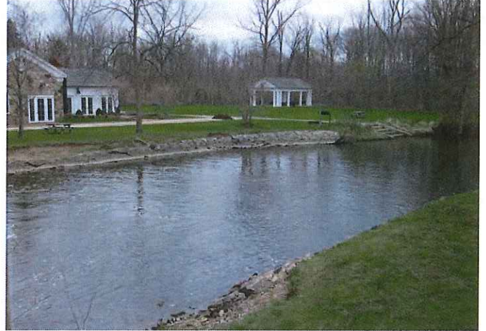
April 27, 2015 Downstream left embankment with grouted rip rap armoring
