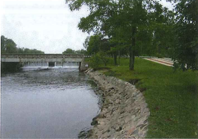
August 27, 2013 Downstream left embankment with grouted rip rap armoring
