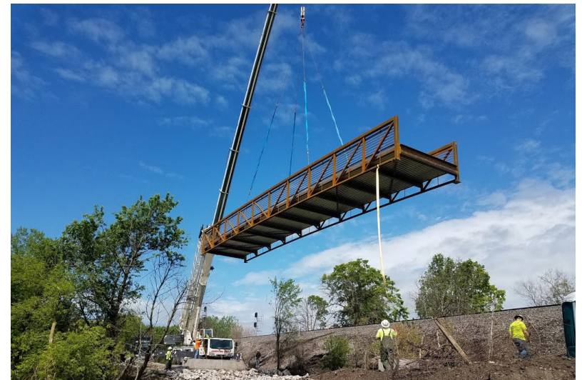
Setting bridge along Border-to-Border Trail in Chelsea area
